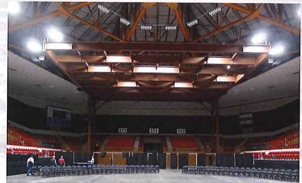
Tony's Pizza Events Center – Salina, Kansas Recently Installed Rigging Structure
